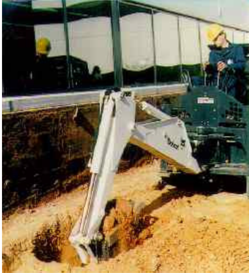
The footing is excavated and exposed prior to installing the piers.
