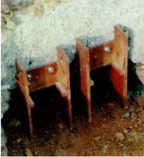
This detail shows ATLAS RESISTANCE PIERS in tandem for 100,000 lbs. support.
