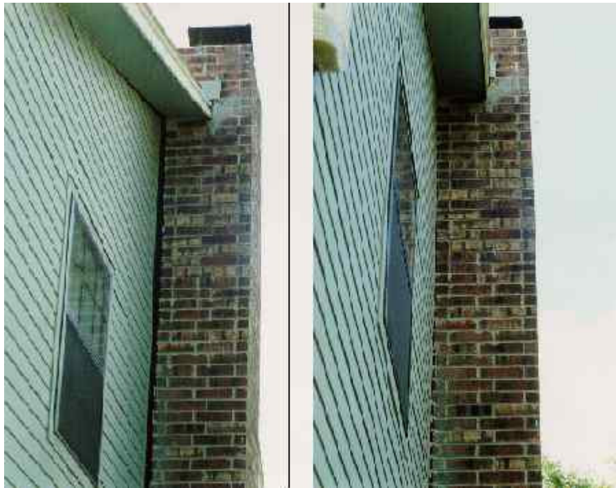
Before Restoration and After Restored with ATLAS RESISTANCE PIERS
