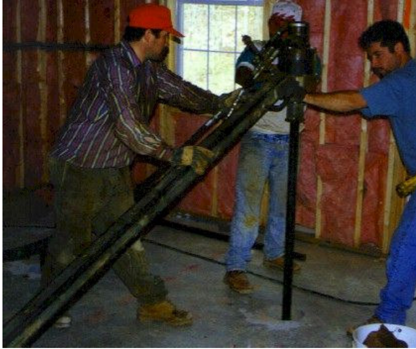
The photograph above shows the technicians installing an ATLAS-Helical Slab Pier at location "P" inside the structure. The pier is installed until the design torque is achieved.
