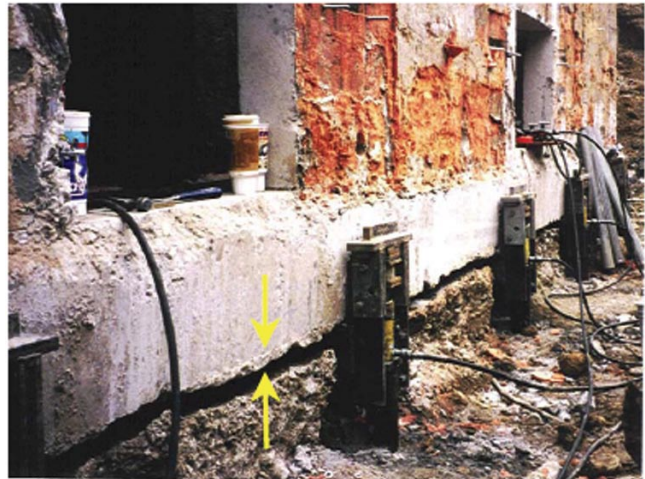
The photographs above show Atlas Resistance® Piers with hydraulic rams attached during the restoration of the structure. Notice the photo at right shows a lift of over 2 inches at the window well.
